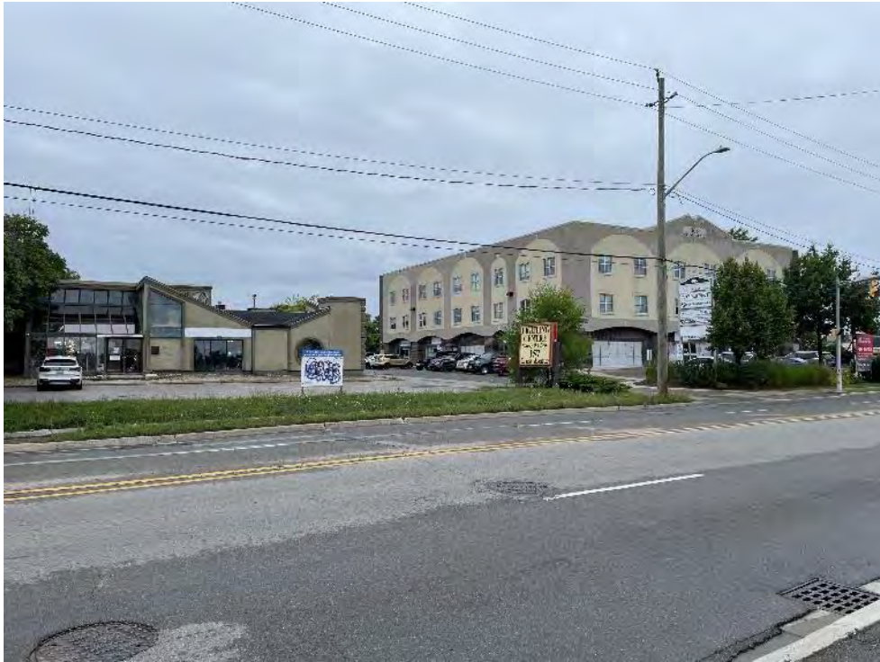
Photo 3: Frontage of the Site buildings at 157 and 165 Cross Avenue, facing north.
