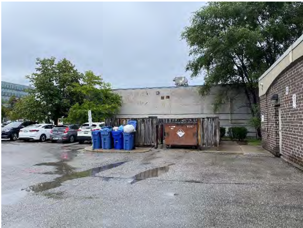
Photo 4: Waste storage area at the back of the Site building at 165 Cross Avenue, facing east. One (1) transformer is in the wooden shed of the waste storage area. Based on the year of Site redevelopment in 2008, it is unlikely to contain PCBs.
