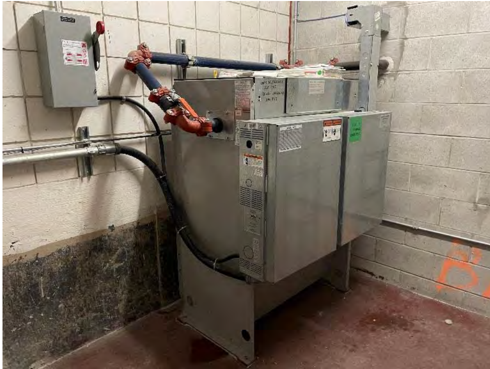
Photo 5: The hydraulic oil AST at the back of the Site building at 165 Cross Avenue, used for the elevator, no leaks have been reported.
