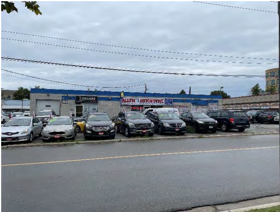
Photo 17: The property located at 570 Argus Road, approximately 50 m east, is occupied by All Fix Automotive.
