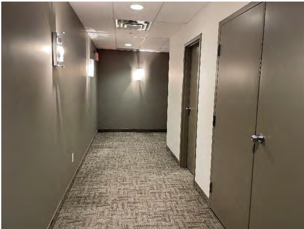
Photo 8: Interior of office space on the second floor of the Site building at 165 Cross Avenue.
